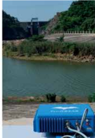
Water reservoir dam
